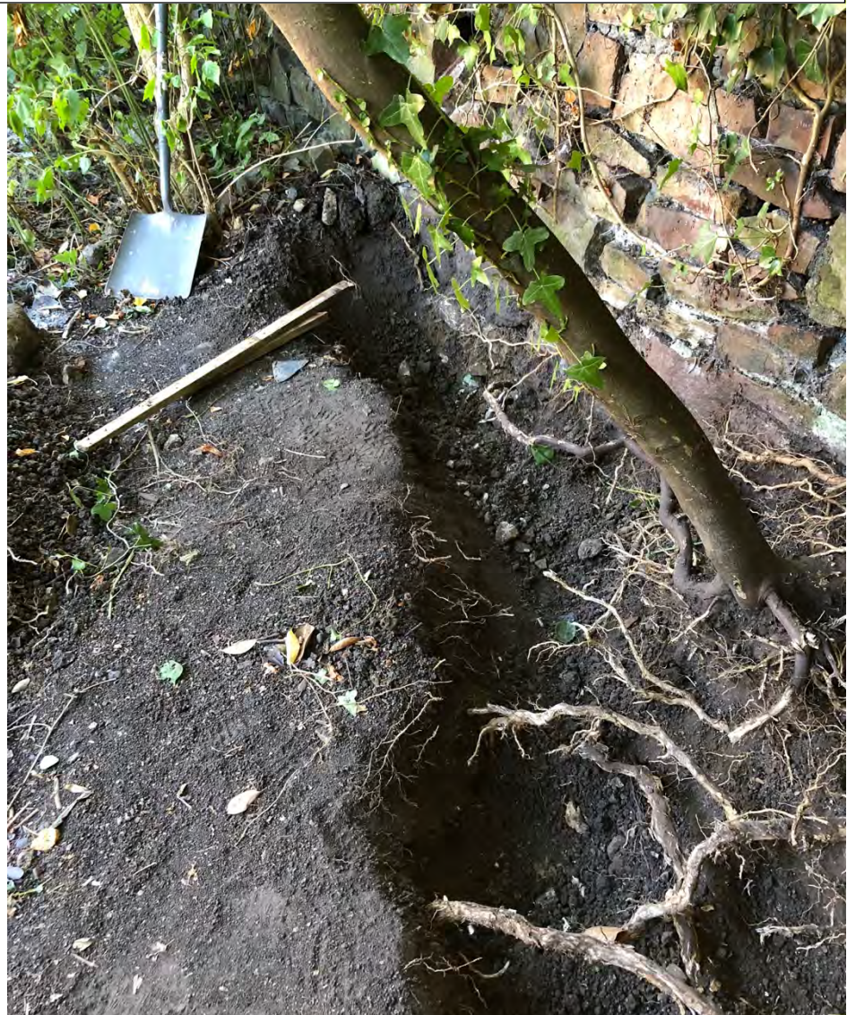
Excavation trench showing roots of 2 small shrubs on the applicants side of the wall
