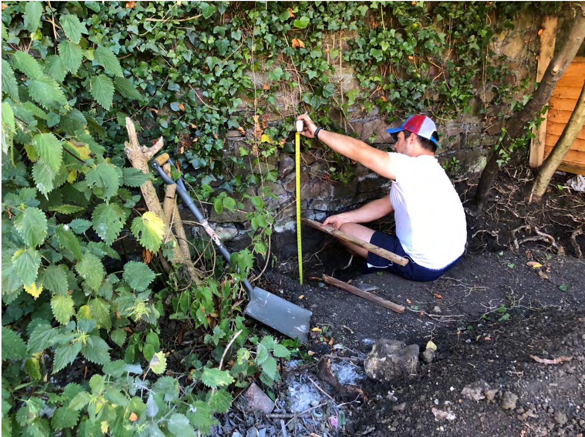
Distance shot of tradesman and excavation on completion
