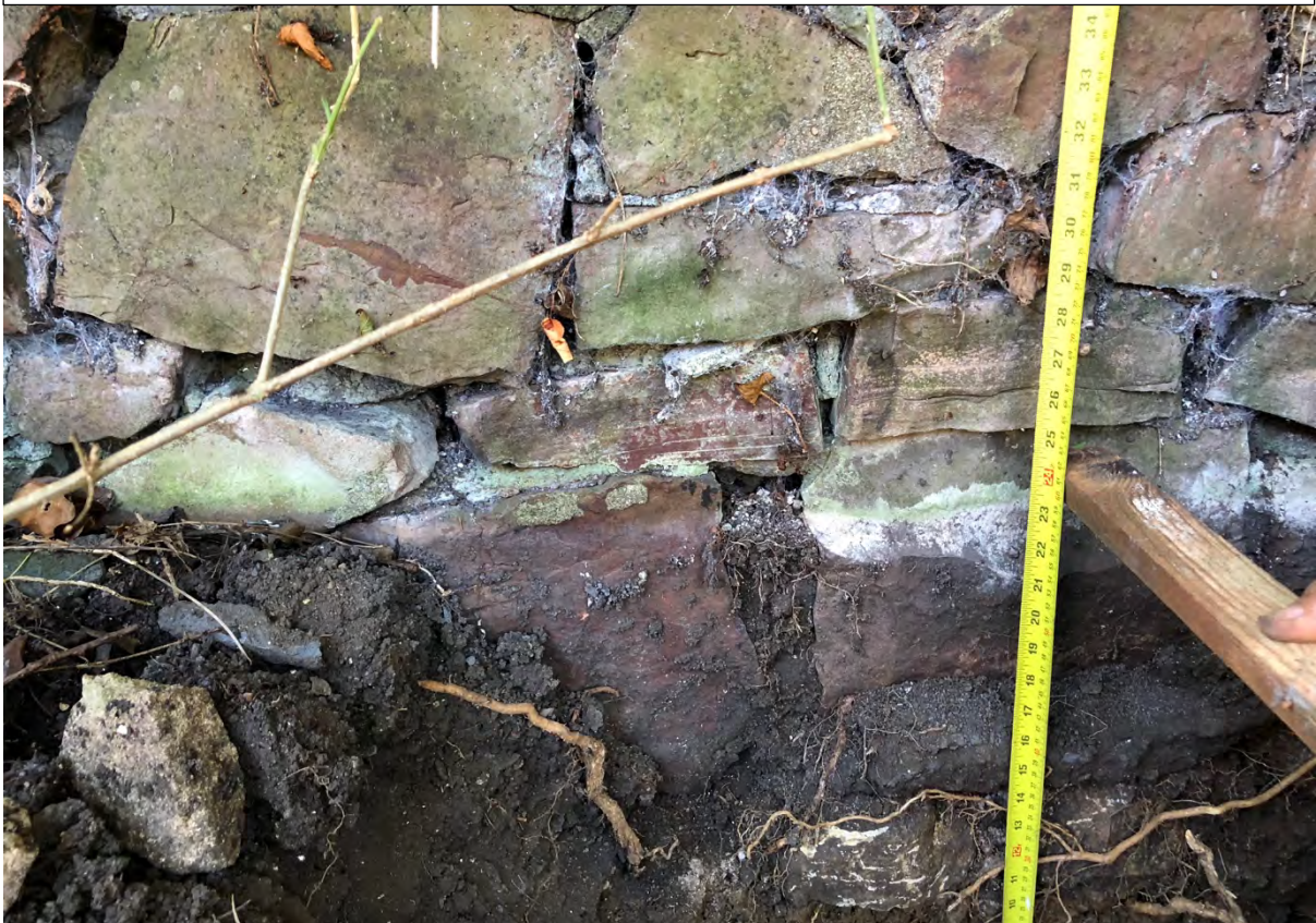
Confirmation that the trench was dug to 600mm depth
