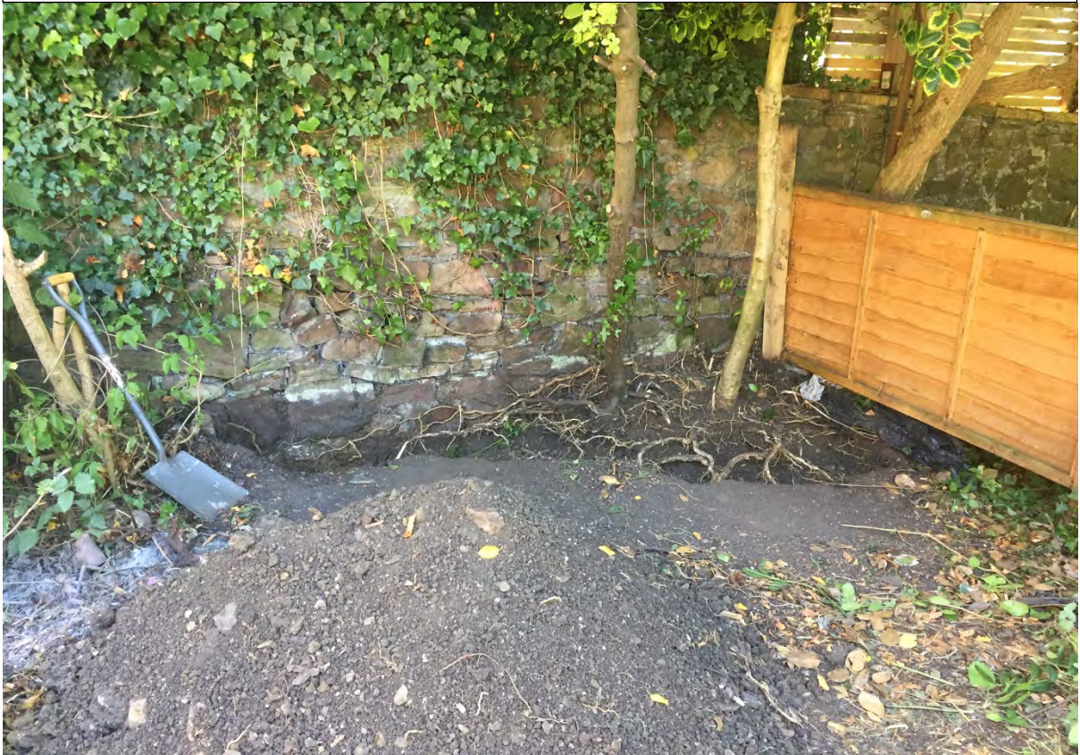
Excavation trench dug in rear garden of No.6 Cotham Lawn Road
